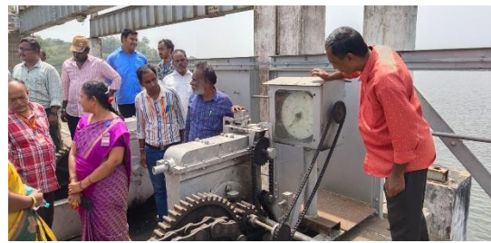
Dial gauge for measuring the depth of flow
