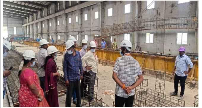
Precast Column under process
