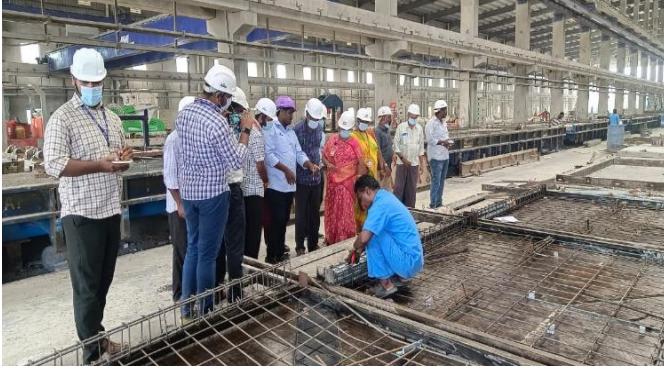
Precast Beam under process
